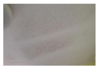
condensation problem, not a roof leak.
