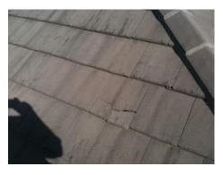
First thing to look for is always a broken tile. Even if the roof is not particularly old, a tile can crack. A tile can have a hairline crack in it that expands with temperature change, or a bird can drop a stone, or an aerial guy could have just been up there and broken one or two tiles. A broken tile will generally be a pretty noticeable leak!
