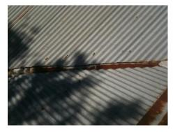
If a valley is rusted through it will leak. If it is blocked with leaves or a tiles has slipped in causing it to be partially blocked, it can leak. You can get clips that hold the little cut tiles in a valley in place to stop them from sliding out, or again, for a temporary fix, use a dab of silicone to hold it there.
