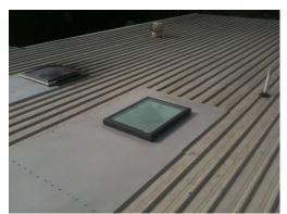
to be at a minimum of 15 degrees pitch or the skylight seal itself will leak (Velux FCM Model is the exception).
