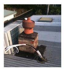
Most of the time the way to fix these leaks is to replace the flashings or install a "Backtray (Drypan) type flashing behind to ensure the lap in the sheets is completely sealed to the top so no water can get into the underlapping pan.
