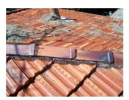
If the mortar around the ridge capping is in poor condition (called pointing), that can leak. Particularly on the ridge if it is coming away and water is getting between the cap and the pointing. The solution here is to repoint (and re-bed if needed) the ridge capping.
