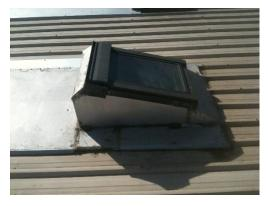
Skylights are first on the list. They leak for all manner of reasons but usually because of incorrect installation. Skylights are generally quite wide and therefore a lot of water will run into the back and need to be channelled around. The flashing work must be perfect.
