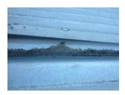
This is pretty simple and obvious to any roofer. Every type of roof sheeting has a minimum pitch that it can be installed at and still work.
