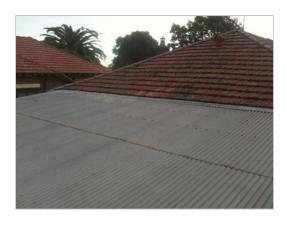
If an end lap must be done, it should lap at least 300-400mm and 2 complete lines of silicone are needed. If there is not enough lap, or gaps in the seal, it will leak.
