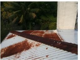
Usually surface rust is not too much of a problem but if the rust is blistering or pitted, this is bad. Zincalume and Colorbond sheets deteriorate very fast once they start to rust, but often they will just have isolated rusting such as in the lap of the sheet.
